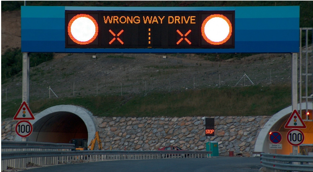
Figure 4: Variable message sign with a message warning drivers about an ongoing incident of wrong way drive.
